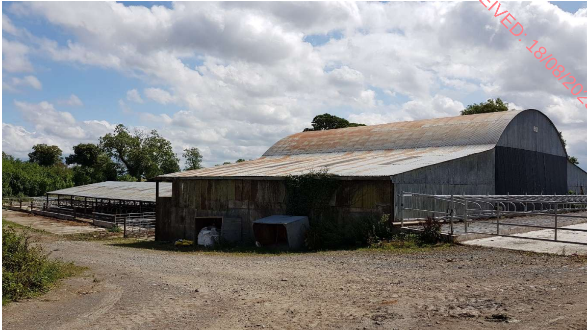
Plate 13.3. Structure 1 looking northwest.
