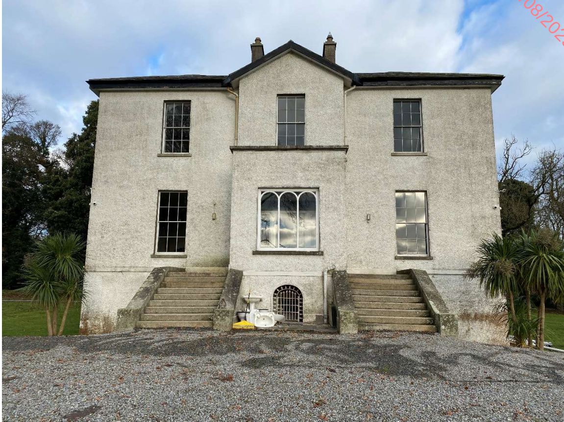
Plate 13.1. Kilree House looking northeast.
